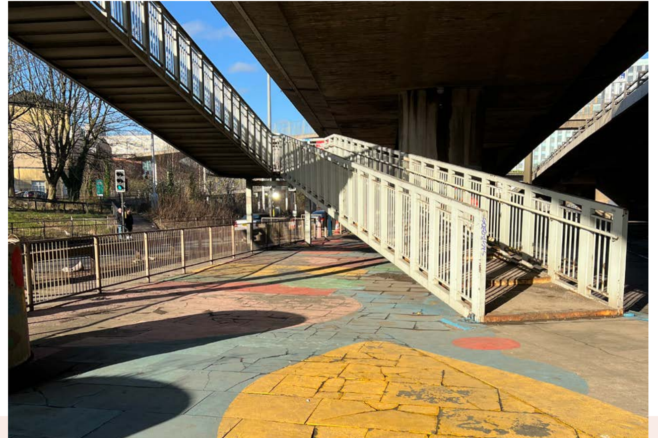
Thermoplastic markings can add some vibrancy to an otherwise dull public space.
