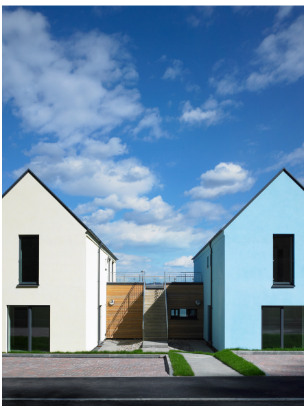
△ Entrance stair to upper flat with front doors to house and lower flat either side
