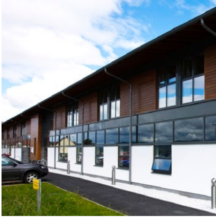
^ Front elevation of Migdale hospital, overlooking the Kyle of Sutherland Image credit: John Paul Photography
