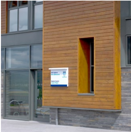
^ Caithness stone and Scottlarch cladding at the entrance of the hospital Image credit: John Paul Photography
