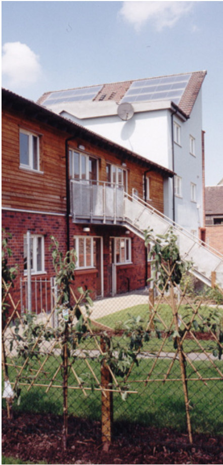
^ Solar water panels located on south-facing roofs
