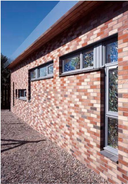
^ Rear elevation - reclaimed bricks and recycled glass windows
