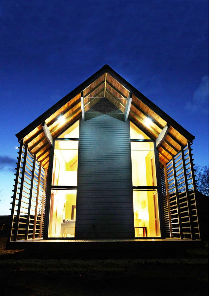
The house was designed to the German 'PassivHaus' standard, whereby houses are designed with a high thermal performance and exceptional air-tightness to minimise heating demand. All elements that make up the building fabric – walls, roof and floor – are designed to be below a U-Value of 0.15W/m²K and an air tightness of 0.6 m³/(h.m²) @ 50Pa.
